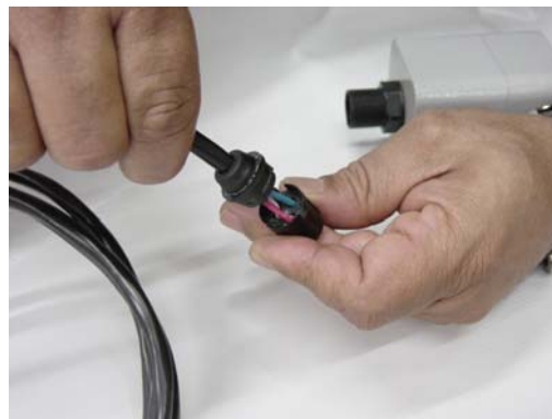
Fig. 1.22 – Inserting the wires in the connector.
