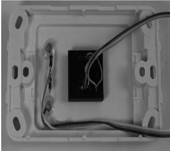
Figure 14-14. ID-12 module mounted behind a blank electrical wall plate
