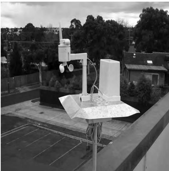
Figure 13-1. La Crosse weather station installed on a roof
