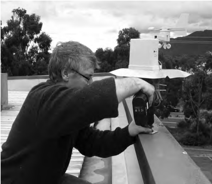
Figure 13-2. Weather station sensors and transmitter being installed
