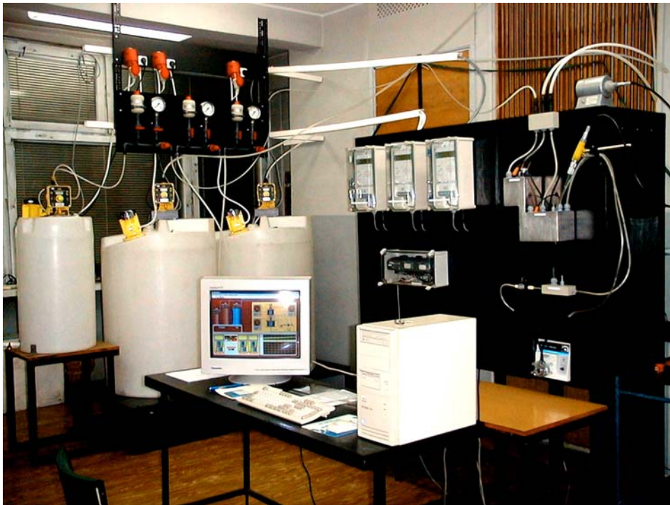
Fig. 2. View of the pilot installation.
