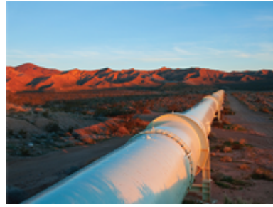
Pipeline Leak and Corrosion Detection
