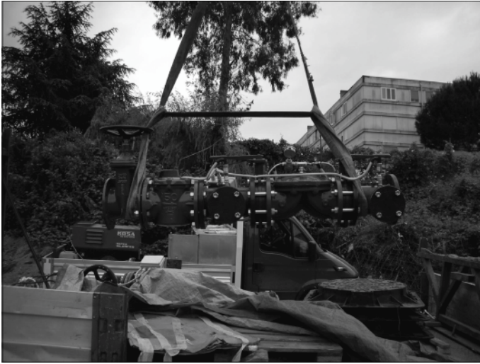
Figure 12. Stage of installation of devices a)
