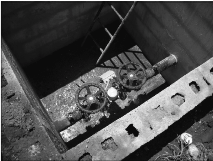
Figure 13. Stage of installation of devices b)
